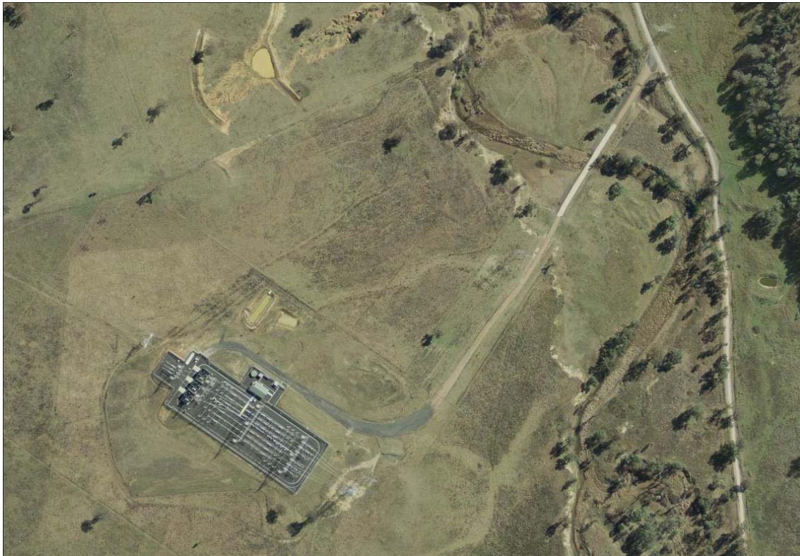
Figure 8-20 Existing substation access road (Ontoit, 2018).
