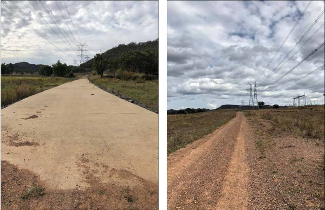
Figure 8-21 Existing Wollar substation access road.
