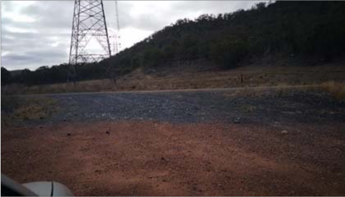
Figure 8-23 Existing substation access road intersection with Barigan Road (Ontoit, 2018).
