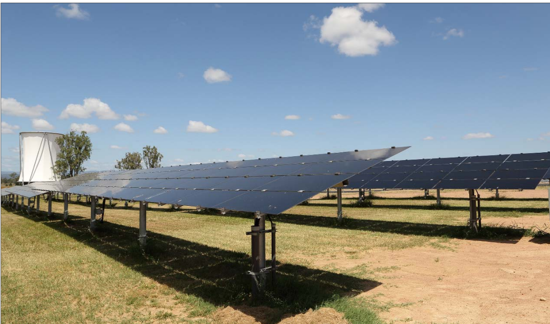
Figure 4-3 Typical single-axis tracking system.
