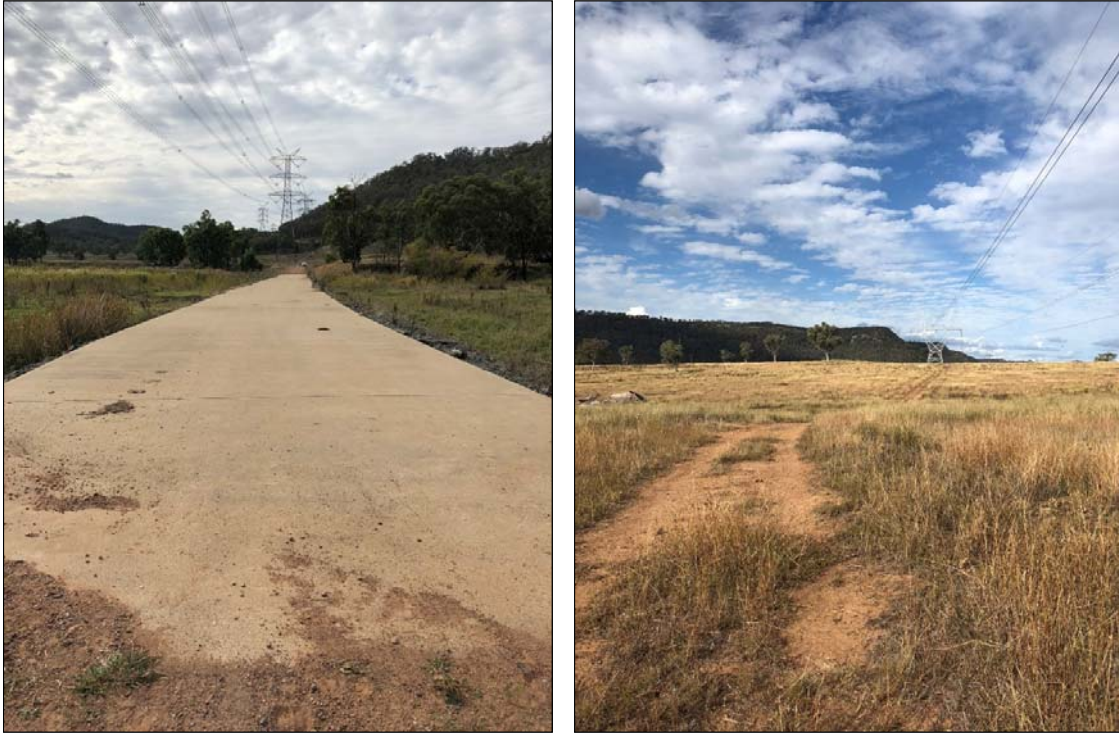
Figure 4-9 Wollar Creek causeway along existing TransGrid access (left) and 330kV TransGrid transmission line between Wollar substation and proposed new substation location (right).
