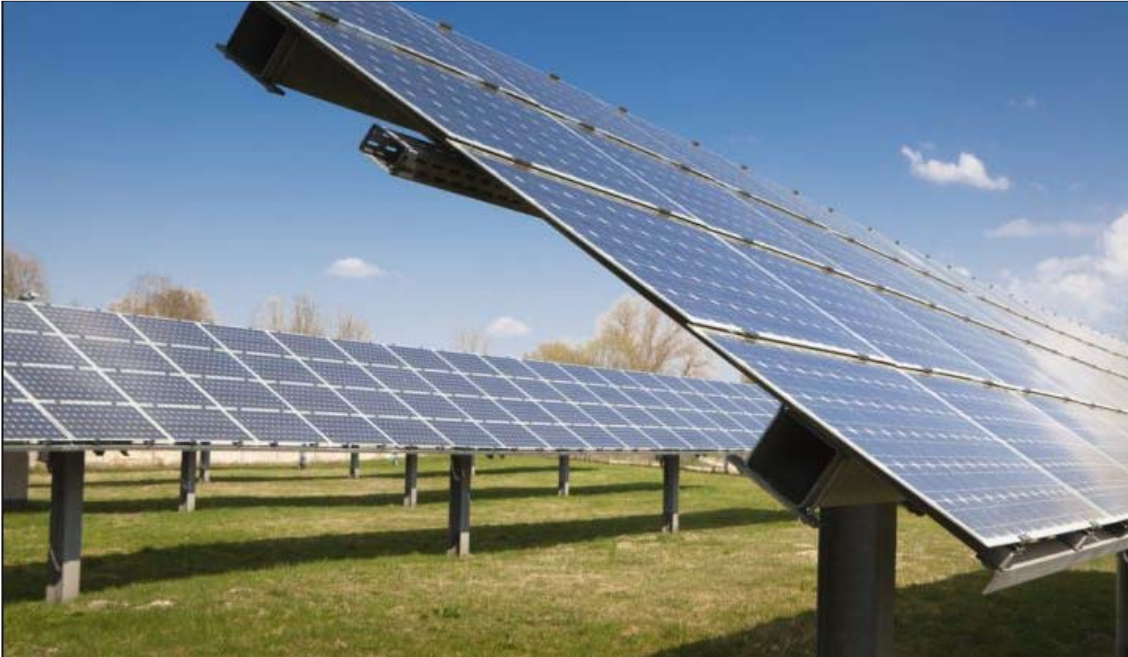
Figure 4-2 Typical fixed tilted system.
