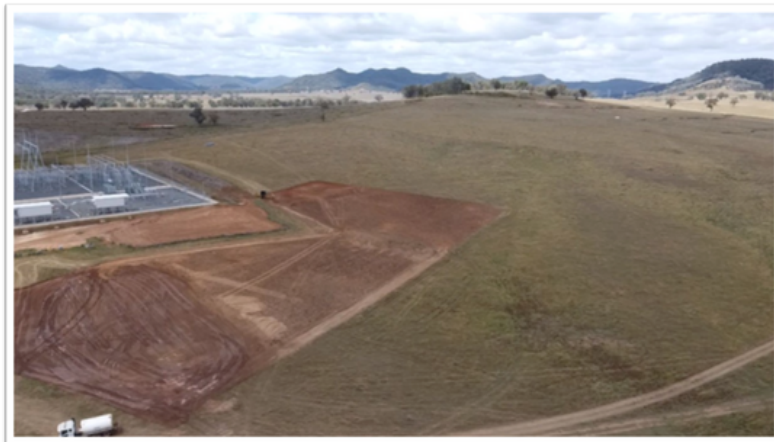
This is a great photo of the initial top soil removal for one of the lay down areas, the civil team brought in material to compact this area so that it will withstand the daily pressures of many semi-trailers delivering solar panels, steel structures and drums of electrical cable.
