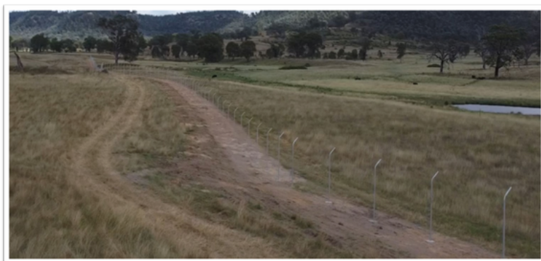
This is a great photo of the initial top soil removal for one of the lay down areas, the civil team brought in material to compact this area so that it will withstand the daily pressures of many semi-trailers delivering solar panels, steel structures and drums of electrical cable.
