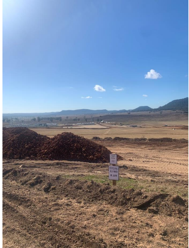
Photo 13: From near eastern boundary looking back towards site compound and substation
