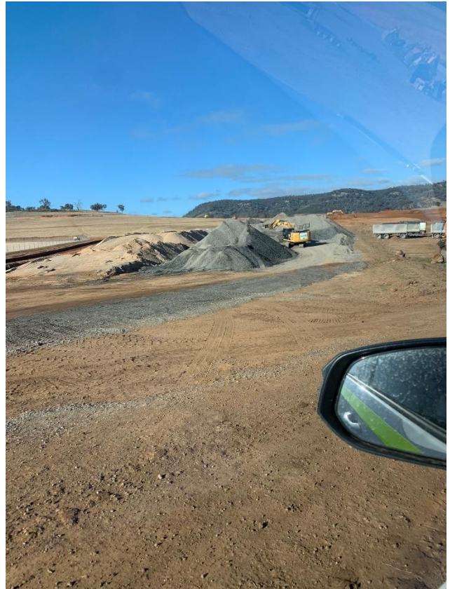
Photo 5: Materials stockpiling area
