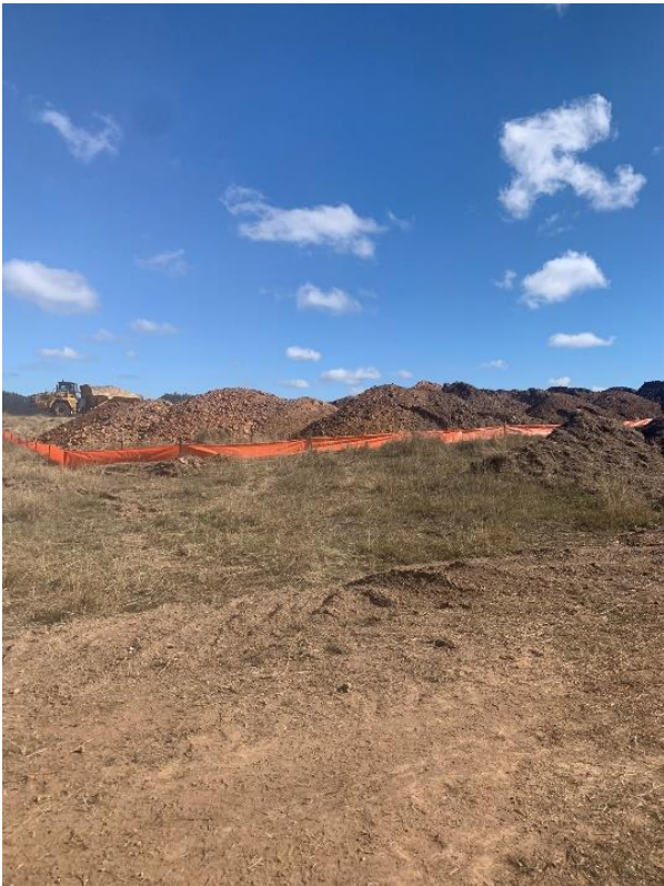
Photo 10: Example of erosion and sediment controls around stockpiling
