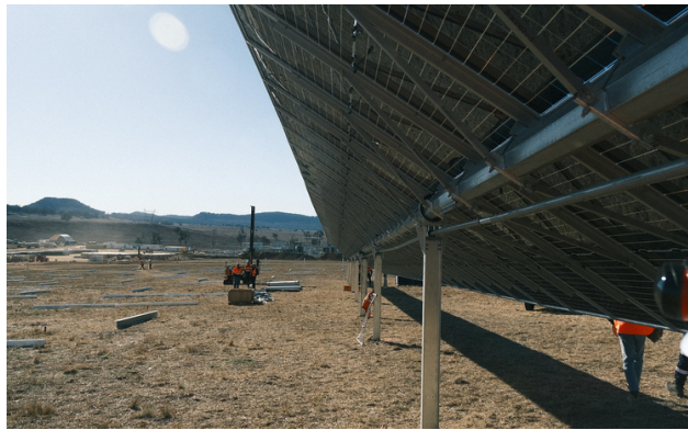
Wollar Solar Farm uses state-of-the-art bifacial modules that can capture energy reflected off the ground and other modules
