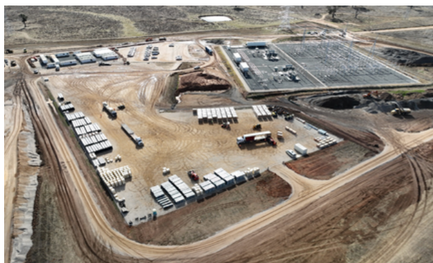
Flyover of the construction compound and newly constructed substation
